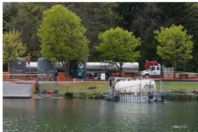
Three on-shore alum storage tanks are being filled from tanker trucks in the background. On the water, there is a barge with alum distribution tanks and lines.
